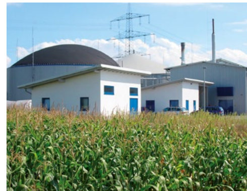
Biomasse-Anlage in Neuried
